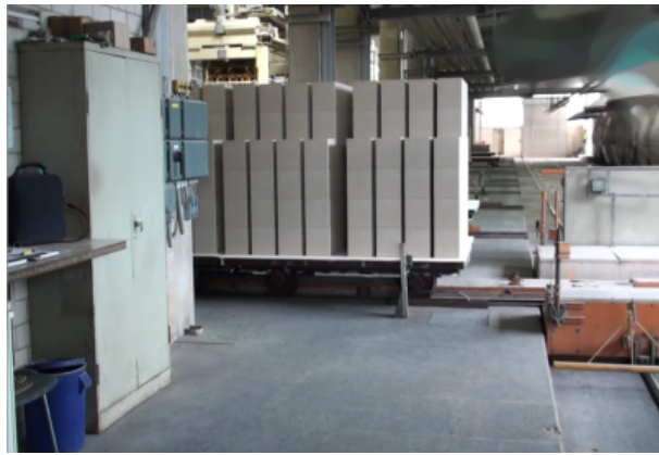
Placing the green cake on the hardening car and drive it in the autoclave.
