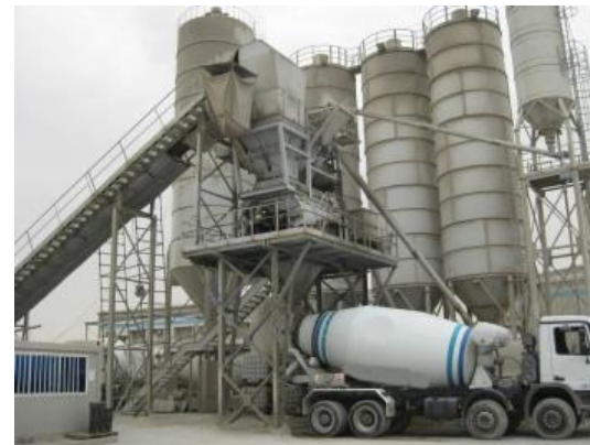
Concrete mixing plant single line
